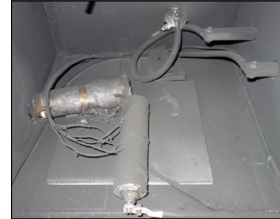
3 mΩ short-circuit on VES140
