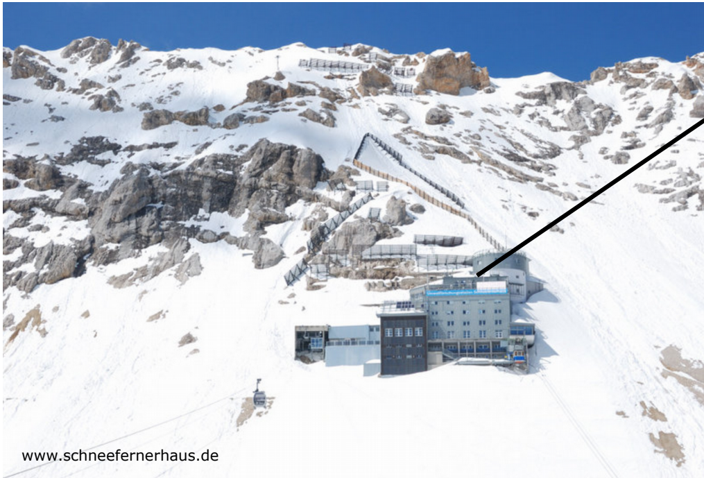
Environmental Research Station Schneefernerhaus – Zugspitze (Germany)
