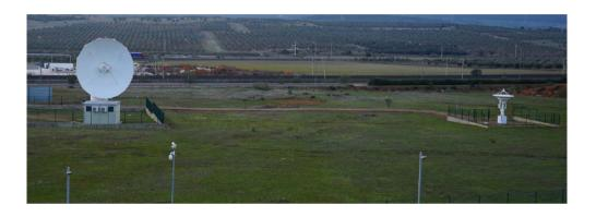
Reduce the antenna mass, example: PL-01: 10,2m/55tons vs PL-03: 11m/18tons Price also divided by 2
