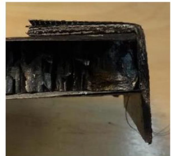
Outer cleat samples setup; delamination at cleat edges before bondline failed
