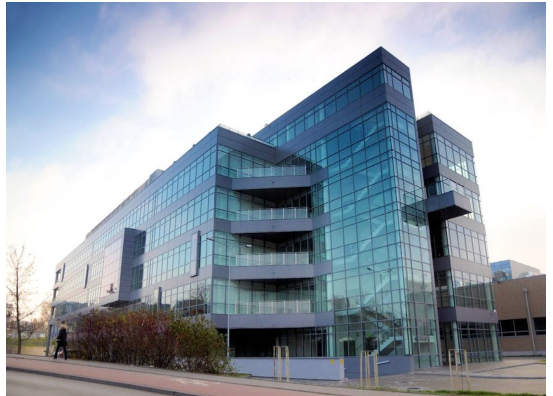
Gdańsk Science and Technology Park - headquarters
