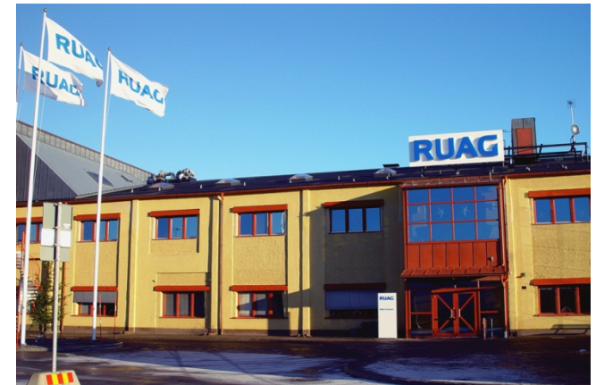
Mechanical systems Linköping operations, Sweden
