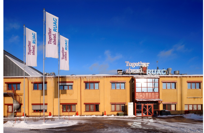
Mechanical systems Linköping operations, Sweden
